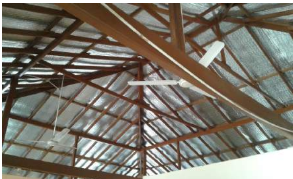
New roofs were paid for by IAHV UK
