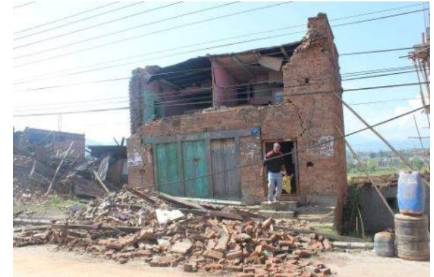
Housing ruined by the Earthquake
